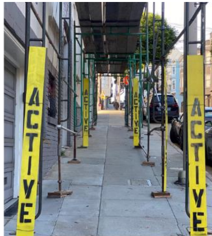
Pedestrian walkways scaffolds
