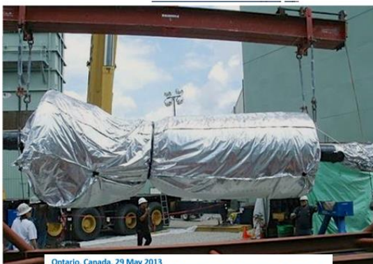
Ontario, Canada, 29 May 2013 A rotor was dropped last week as it was unloaded at new power generation facility in Durham Ontario, Canada
