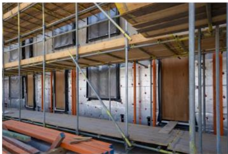
Independent access scaffolds with pavement lift
