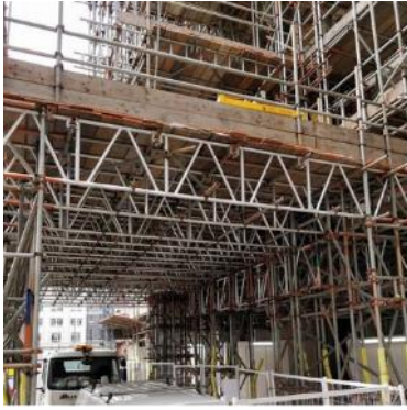
Pavement gantry scaffolds
