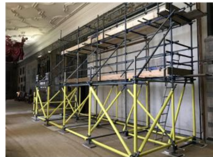
Independent access scaffolds with bridge spanning up to 6m
