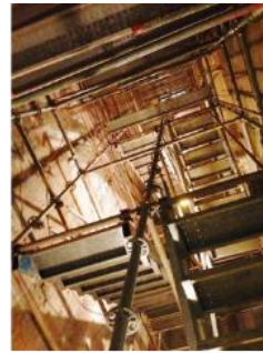
Lift shaft scaffolds
